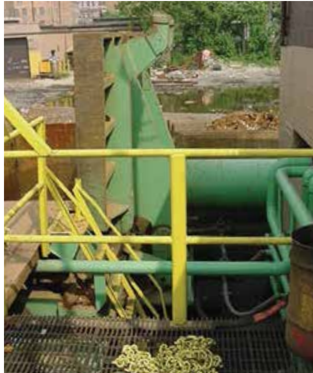
Left and right image: D&J Model 410 baler installed at SCA's Courtland Avenue yard in Chicago.
