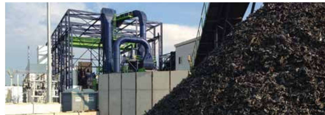
Wendt Corporation Model 130 HEAVY shredder installation at Camden Iron & Metal in Camden, NJ.
