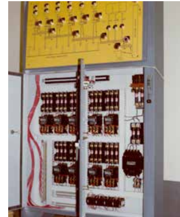
Top and middle image: Electrical control panel that Thomas Wendt assembled and wired in the garage of his family home on Fairmont Avenue.
