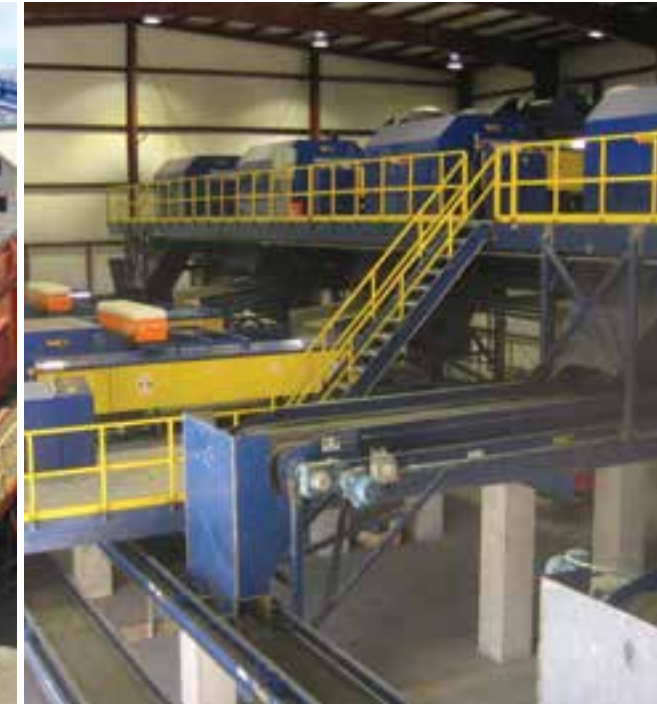
Outside view of the first fully- integrated wire recovery plant at Western Metals in Plymouth, UT.
