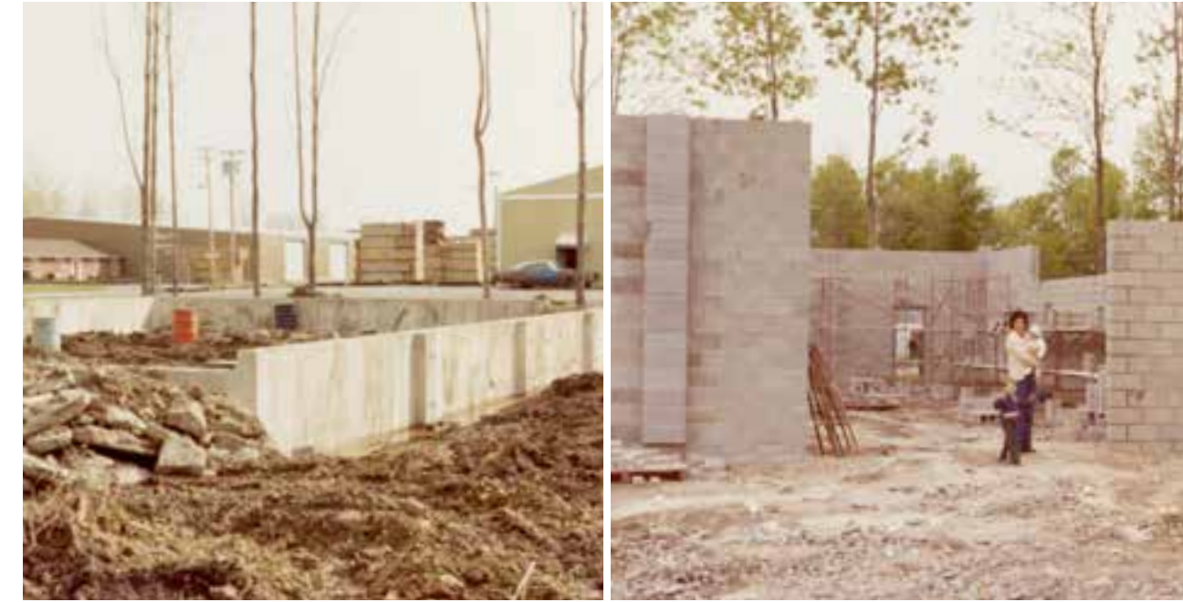
Top left image: The foundations have been poured during this early stage of building the Industrial Drive plant – (Phase I).
