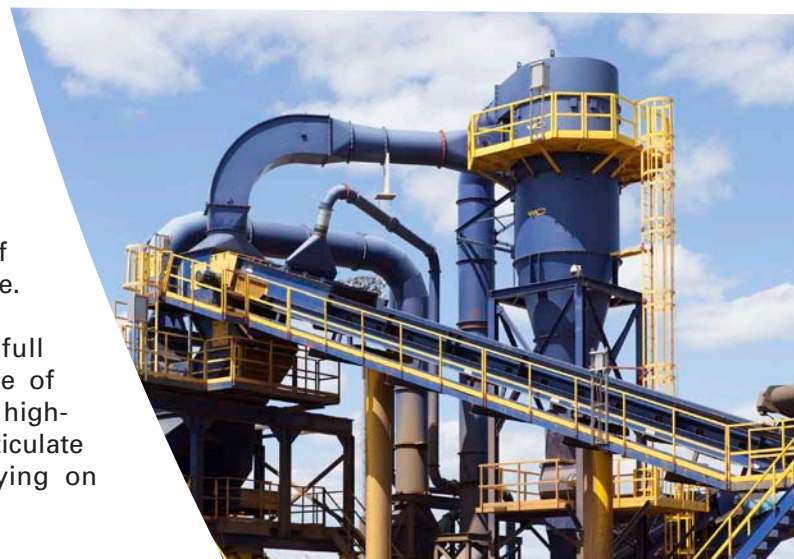
Z-Box and Air System
