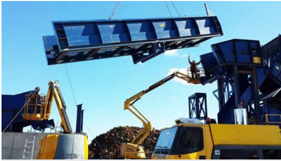
WENDT M6090 Shredder Installation
